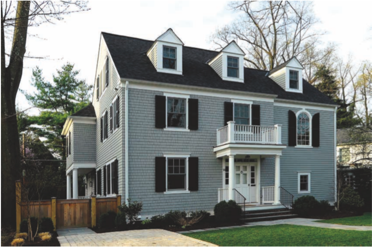
GTM Architects designed the Abells' new home to reflect the architectural styles of other houses on the Chevy Chase Village street.
